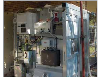
Exeloo Euro Kit Structure with all electrical & plumbing fittings in place
